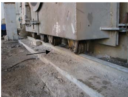
Door rails on the floor in front of the kiln hood.
