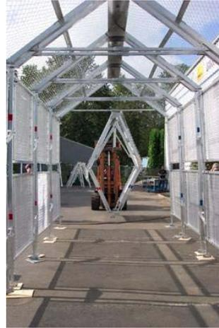
tunnel had to be tall enough to set up close to the coating to reduce the momentum force generated by distance from the coating to the cage. In addition the tunnel had to be wide enough and tall enough for mobile equipment like the Brokk tear out machine pass through. This presented a problem in that tunnel for
