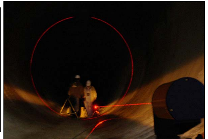
Precision Laser Brick Alignment System
