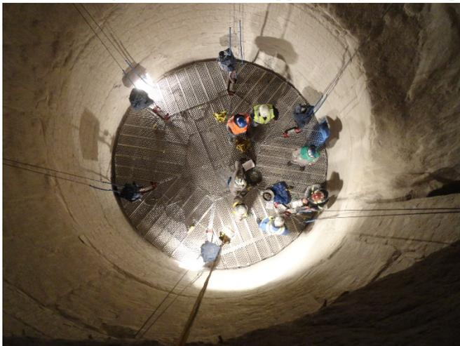
In addition to the increased safety provided by a thorough inspection, the EZ Lift makes routine maintenance safer for the work crew. The platform boasts one of the highest safety ratings in the industry and meets OSHA, ANSI, CSA and EN safety standards. Maintenance repairs are also much safer and more efficient because the necessary materials and equipment are stored right on the platform, eliminating the danger associated with manually moving materials up and down scaffolding systems.
