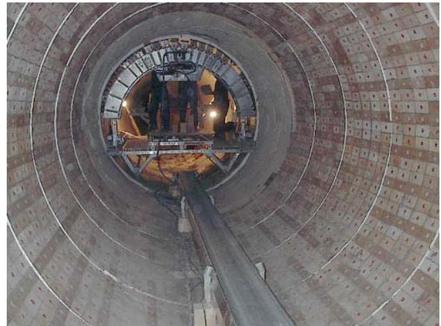
After having used the belt conveyor for the first time, the plant personnel commented that the number of damaged brick had decreased to almost nil. Compared to the old method using wheelbarrows for the transport, the belt conveyor contributed to better installation quality by reducing manhandling of bricks.
