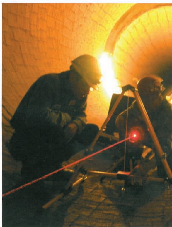
Figure 4. Radialign laser ensures bricks are properly aligned.
