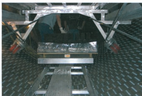
Figure 5. Port-A-Trac system provides consistent brick to masons.
