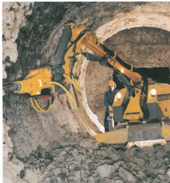
Figure 3. Brokk demolition machine reduces tear out time.
