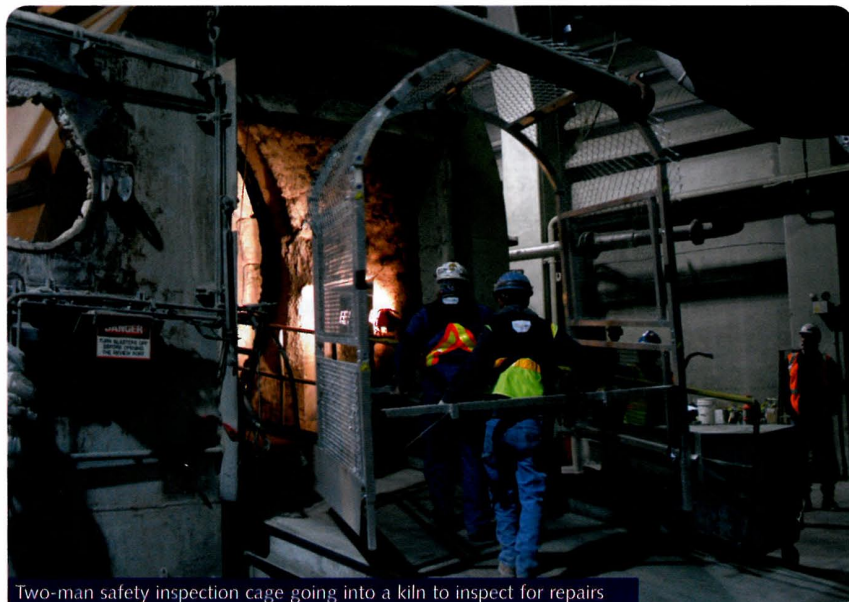
Two-man safety inspection cage going into a kiln to inspect for repairs
