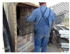
The new kiln came with its own maintenance challenges. The only access point was a 54-inch-high by 36-inch-wide door 80 feet above grade that required a crane to reach with materials and tools. Crews also had a larger continuous area to inspect and service.
