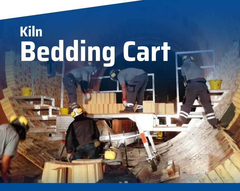
**Speed up bedding out larger kilns** while providing a safe, ergonomic working deck with stairs for higher brick placement.
