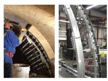
**TWO ARCH SYSTEM** With a two arch system, one row of brick can be keyed while another row of brick has begun on the front arch increasing production time
