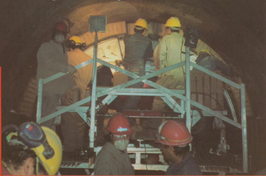
Below: Bricking Solutions bricking machine inside the kiln at Juan Minetti
