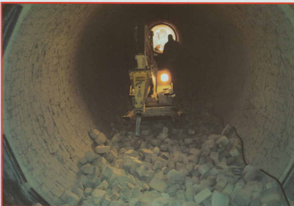
Below: A Brokk tear-out machine at work inside the kiln
