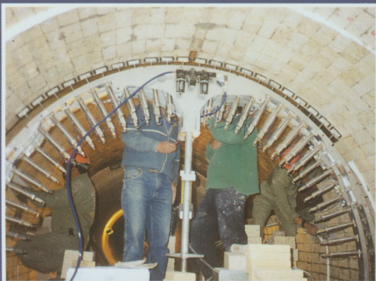
The Bricking Solutions' bricking machine in operation at the CMPC plant, Chile.
