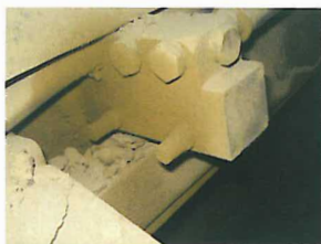
Build-up of dust and mortar.
