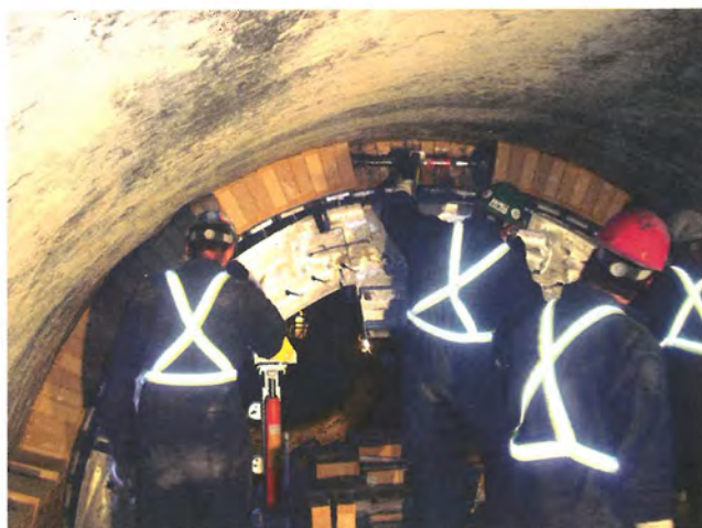
Figure 5. Hydraulic jack in use, used to tighten the ring radially.
