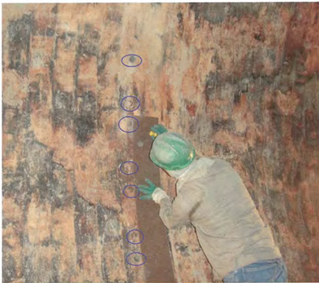
Figure 1. Inaccurate measurement using the welds of the shell as guidelines.
