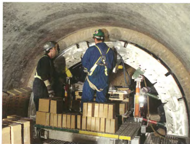
Figure 4. Pneumatic bricking machine with a lightweight aluminium double arch.
