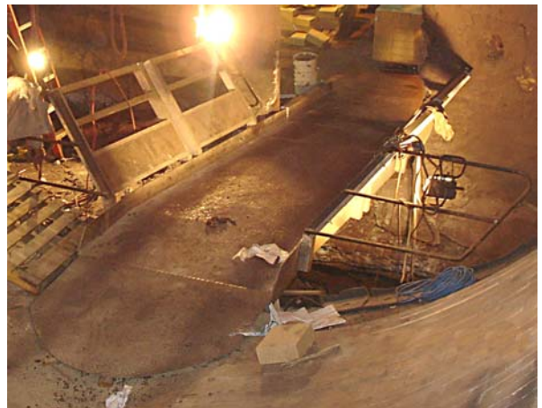
The previously used steel ramp took 3 hours to install and the new lightweight aluminum ramp took 30 minutes.
