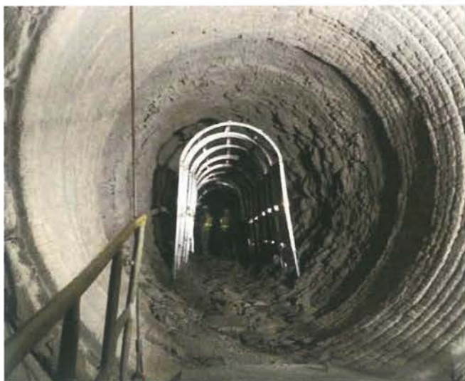
Bricking Solutions' personal protection tunnel withstands impacts of up to 112 kg dropped from 455 mm.
