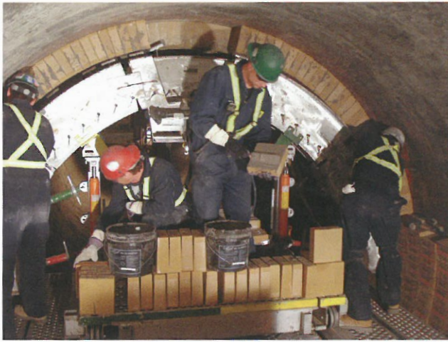
Figure 1. Refractory installation.
